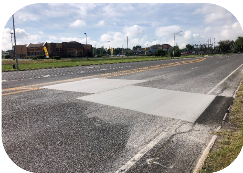
Patching project on N. Seminary Street
